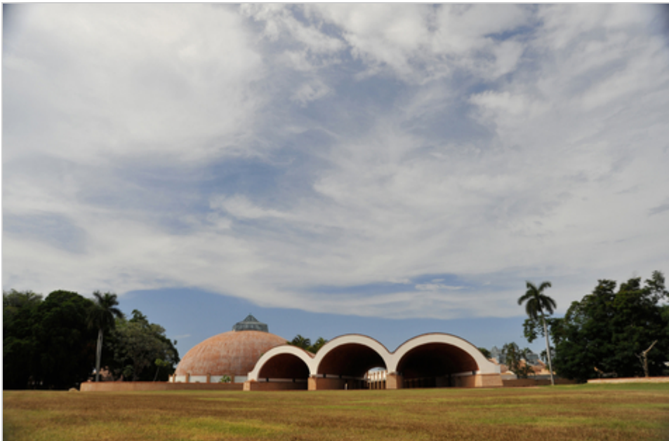
The School of Plastic Arts features swooping Catalan vaults, which are constructed from local brick.
