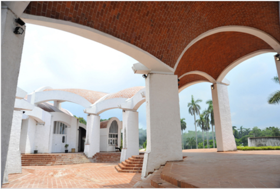
The School of Dance designed by Porro.
